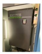
The new ABB 200 (or 400) hp air cooled drive cabinet will be installed within 50 feet of the existing panels. The old Baldor drive will be removed, and customer will store for spare parts or dispose of old drive.
