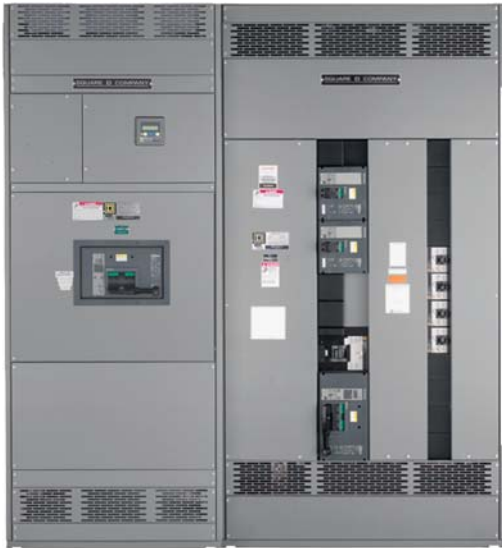
PowerPact™ R-frame Main Circuit Breaker on Left with I-Line™ Distribution Section on Right
