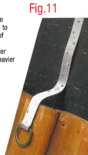
Conform Anchor Leg to the tile profile.
